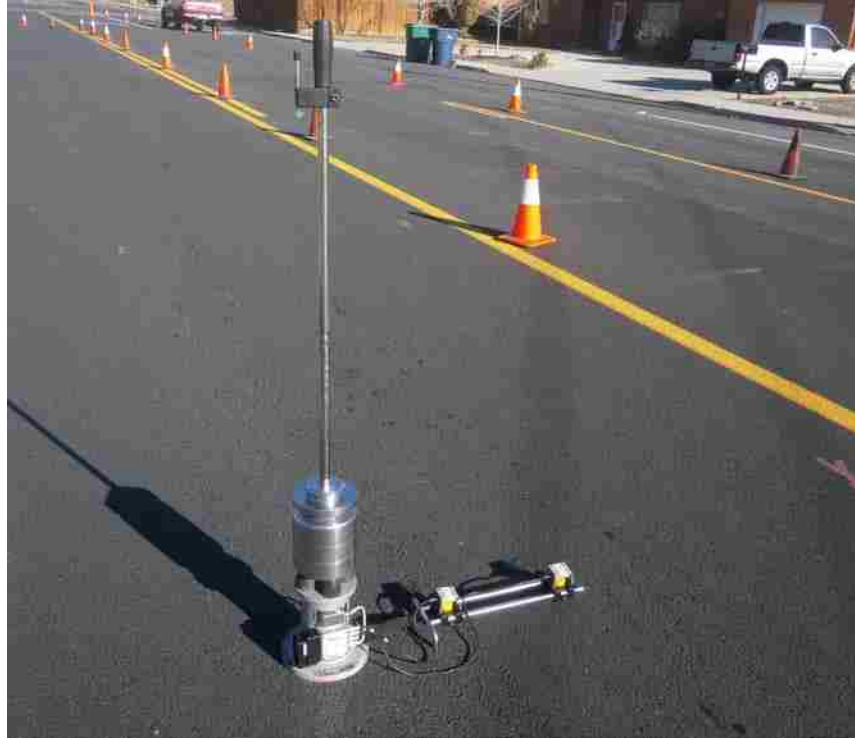
Figure 3-19: PFWD testing of pavement.
