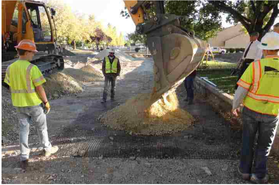
Figure 3-10: Installation of geogrid reinforcement at Springville site.
