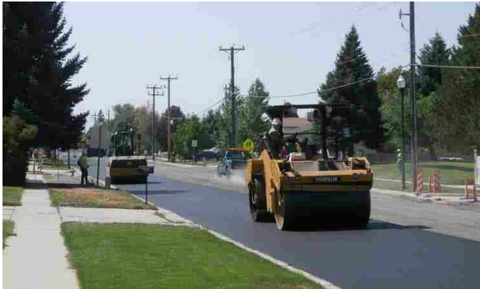
Figure 3-7: Vibratory and finish rollers for compaction of HMA at Orem site.
