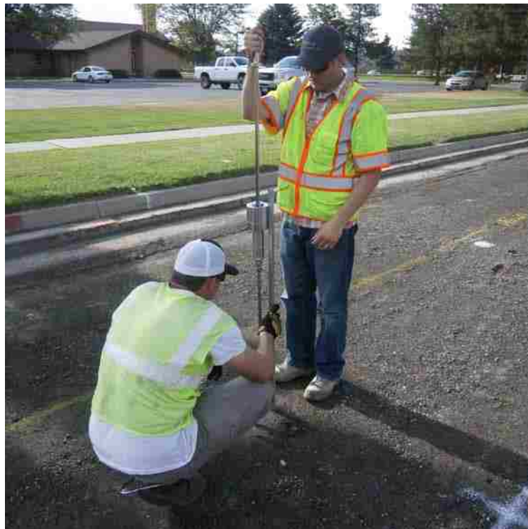
Figure 3-18: DCP testing of base layer.
