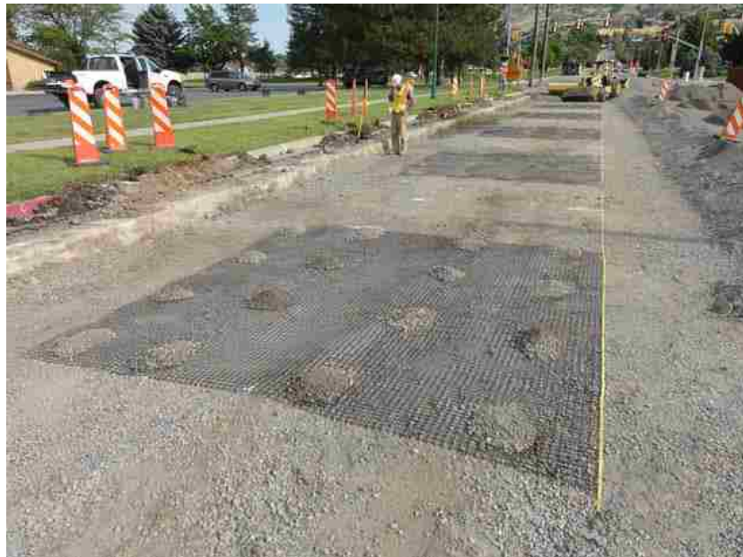
Figure 3-5: Installation of geogrid reinforcement at Orem site.
