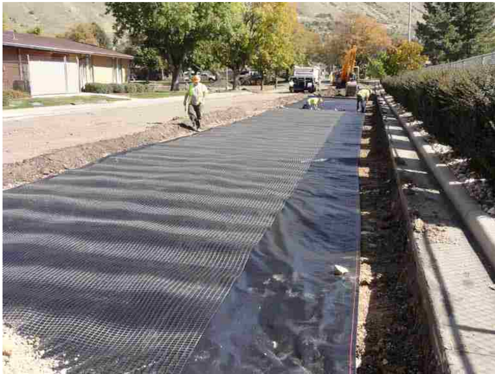
Figure A-3: Installation of geogrid reinforcement at additional Springville site.
