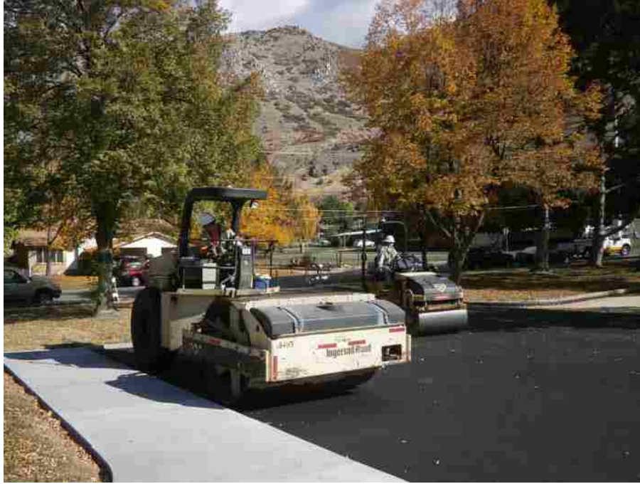
Figure 3-12: Vibratory and finish rollers for compaction of HMA at Springville site.
